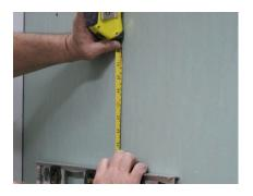
Using a level, mark dimensions of recessed niche onto current substrate.
