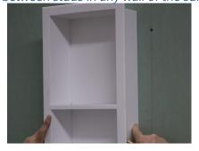
Dry fit panel to ensure that you have 1/8" expansion space between tub deck, shower base and from walls.
