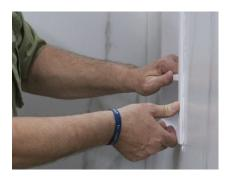
Secure the niche in place with tape. Allow 24 hours for the sealant to dry before use.
